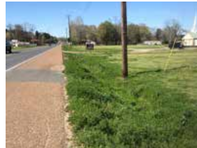
Existing sidewalk conditions U.S. Route 71 Photo Credit: UNO Team
