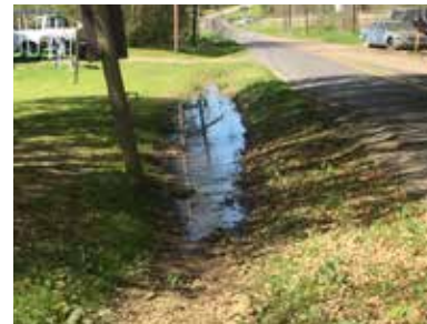
Existing sidewalk conditions on Mill Street Photo Credit: UNO Team
