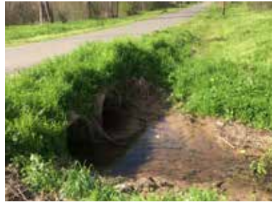
Existing drainage conditions on Lebrum Street Photo Credit: UNO Team
