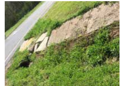
Existing sidewalk conditions on Mill Street Photo Credit: UNO Team
